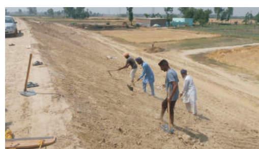
Grading of slopes using Machinery and Manual labour
