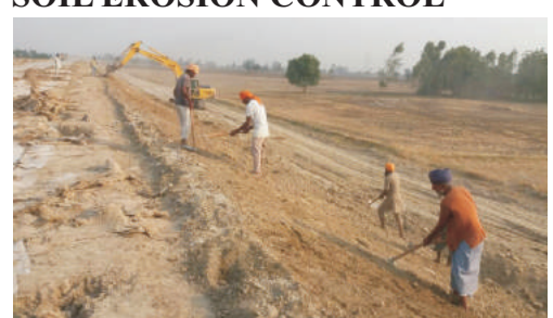
Grading of slopes using Machinery and Manual labour
